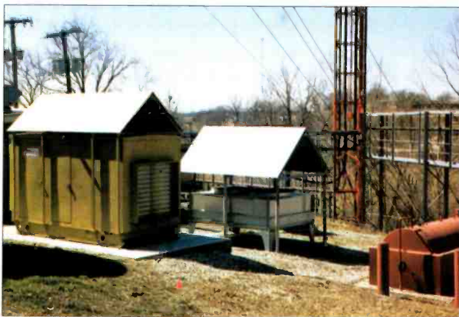
In addition to the tower, there are numerous other items such as outdoor heat exchangers, generators and the generator's fuel supply that all need to be readied for the cold weather ahead.
