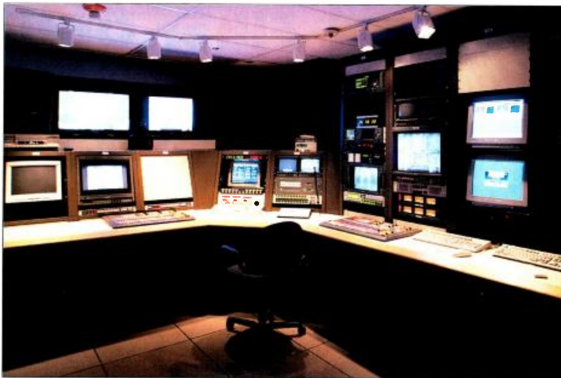
DTV facilities must handle several layers of data, including video, audio, control and metadata, plus legacy analog signals. KHOU, Houston, routes both standard and high-definition signals through its dual master control rooms. Photo courtesy of Tektronix.
